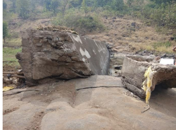
Figure 13: Fragmented condition of CNB (PPCB2)
