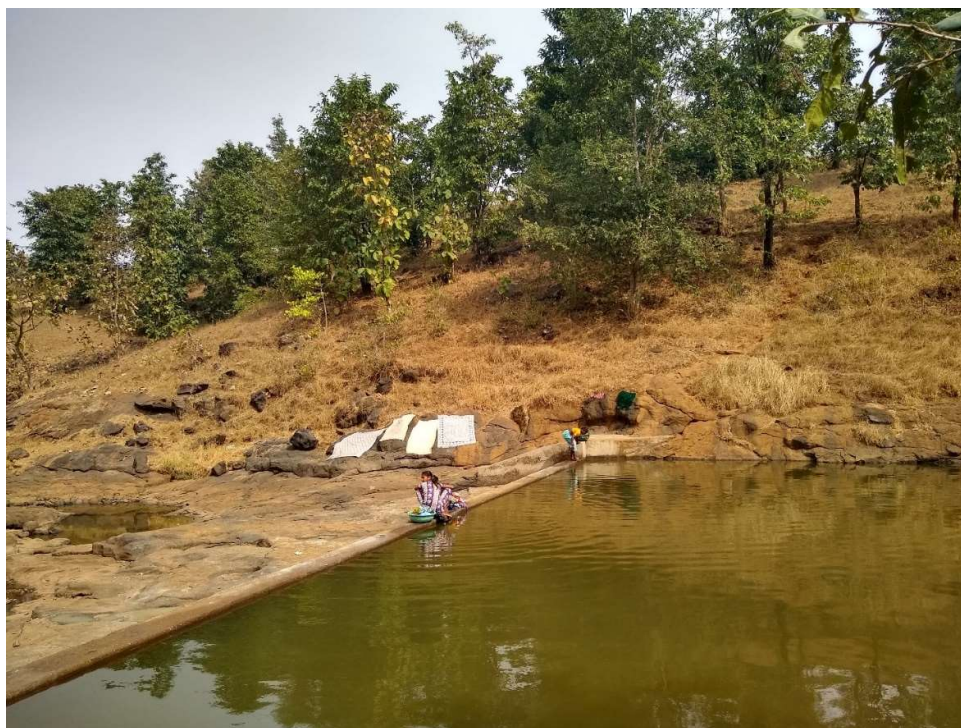
Figure 27: Water levels and condition of Aroehan Bund
