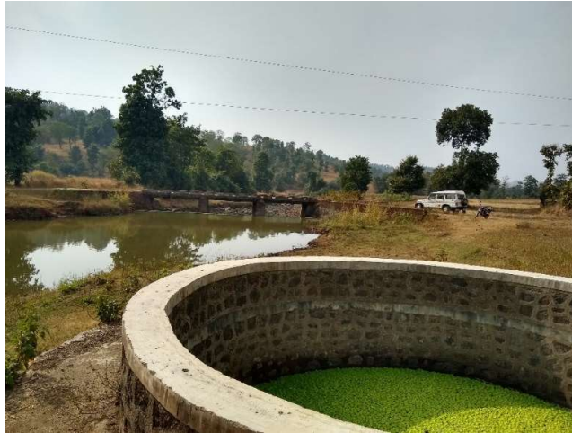
Figure 29: Condition of well 1 containing hyacinth growth
